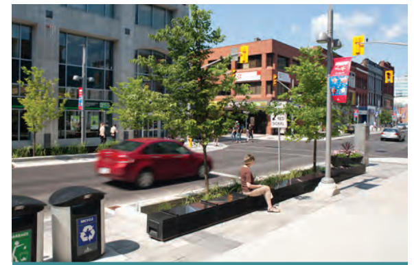
Figure 1.3.2: Bioretention planters are an integral part of Kitchener's new King Street streetscape. They not only help manage stormwater runoff from the road, but they also provide amenity value through street greening and providing pedestrians with a gathering space. (Source: City of Kitchener)
