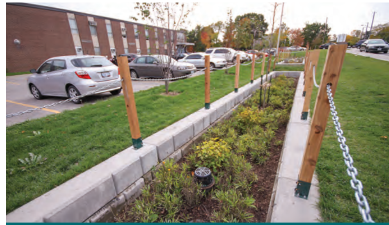
Figure 6.4.11: For bioretention planters with deep, flat-bottomed storage areas, there is more flexibility in placing the overflow spillway because the practice functions as a detention basin, not a conveyance path during infrequent storm events. (Source: CVC)
