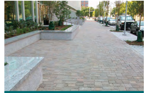
Figure 4.3.24: Permeable paver sidewalk along a minor arterial in Raleigh, NC. (Source: Fred Adams Paving )
