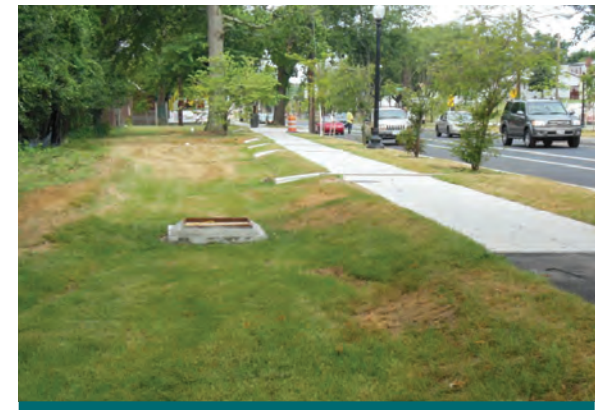
Figure 4.3.20: Grassed bioretention treating road runoff in a wide boulevard space. The grassed bioretention can blend with a corporate property lawn and will be easy for property maintenance staff to maintain with little to no training. (Source: CVC )
