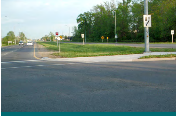
Figure 4.3.26: Major arterial road. (Source: Aquafor Beech)
