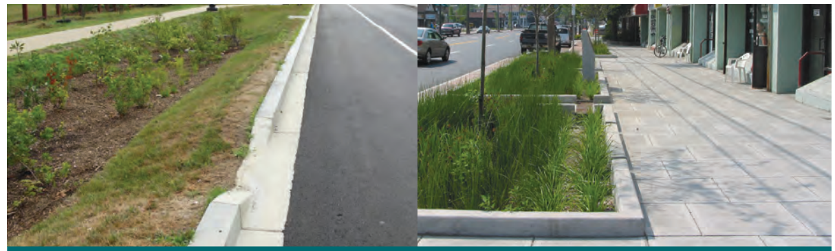
Figure 4.3.23: Boulevard bioretention (left) treating runoff from a minor arterial in Washington, DC. (Source: LID Center). Bioretention planters (right) along a minor arterial in Bridgeport, CT. (Source: Tavella Design Group)
