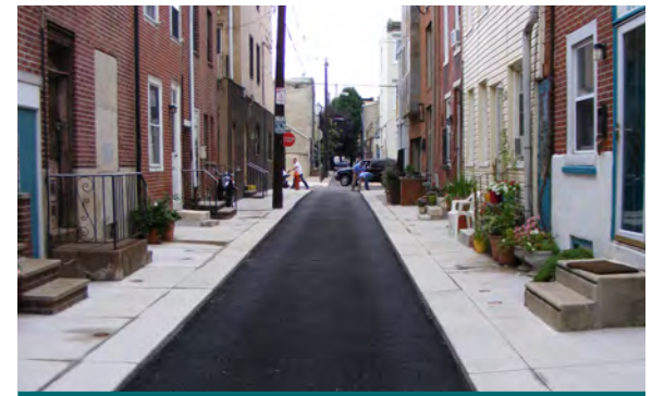
Figure 2.5.1: Porous asphalt and other permeable pavement materials have been used extensively in alleyways and other low-traffic applications in Chicago, IL and Philadelphia, PA (Source: Aquafor Beech)
