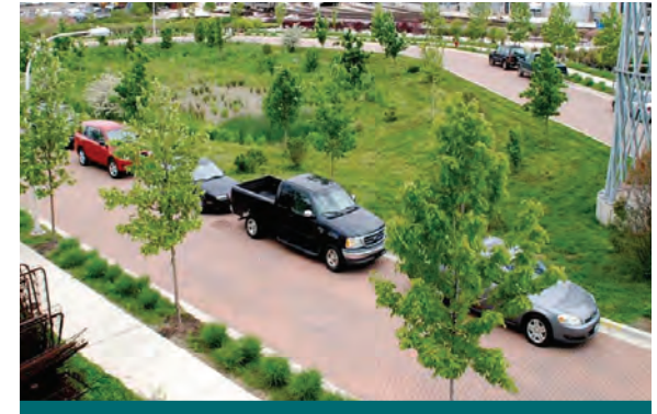
Figure 4.3.16: This light industrial and commercial road in Chicago uses permeable pavers from curb to curb and loops around a dry detention feature. (Source: ICPI)
