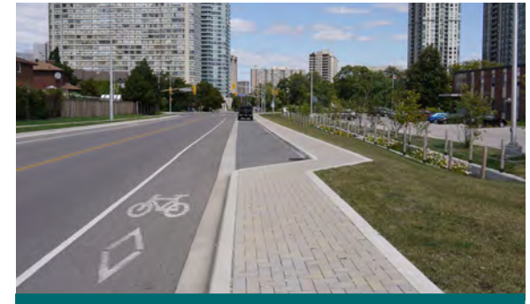
Figure 2.5.4: Permeable pavers can be used to create visual interest within the ROW. On Elm Drive, located in Mississauga, permeable pavers with different shapes and colours were used for parking lay-bys and the sidewalk. (Source: CVC)
