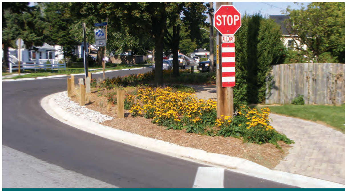
Figure 4.3.35: ROW retrofit opportunity – local parkette and pedestrian crossing improvement. (Source: Aquafor Beech)
