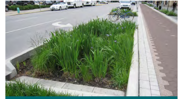
Figure 2.1.4: Bioretention curb extensions can be part of a street reduction, where a lane within the roadway can be dedicated to other uses such as street parking, bicycle lanes, pedestrian crossings, and street greening. (Source: CVC)
