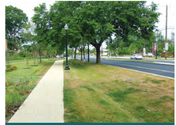
Figure 4.3.19: Enhanced grass swale located between the curb and gutter in Washington, DC. (Source: LID Center)
