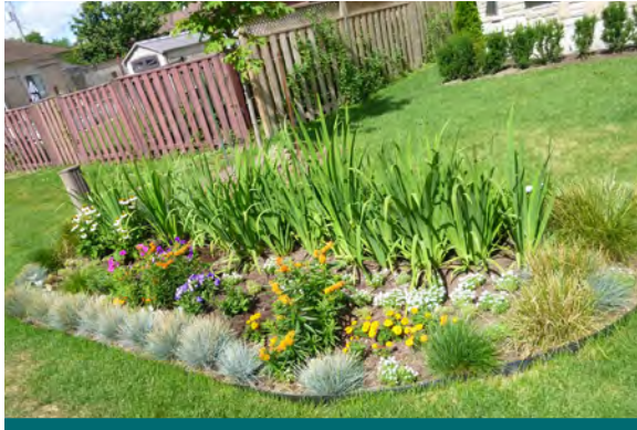
Figure 10.1.1: A photograph showing one the bioretention features in the Lakeview project maintained and even augmented with additional plantings by the homeowner. Private owner maintenance of boulevard bioretention units was found to be a practical approach for the Lakeview project, however, areas where there is a higher occurrence of renters the municipal or hybrid approach may be better suited. (Source: CVC)
