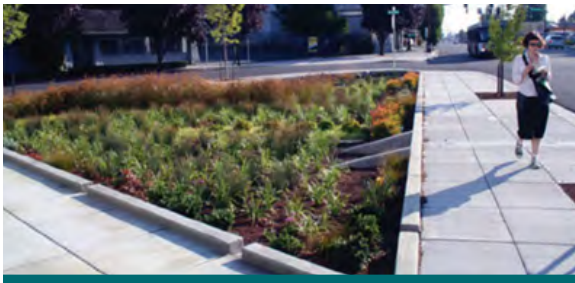
Figure 4.3.27: This large bioretention planter along an urban arterial replaced a large unused expanse of asphalt. (Source: Nevue Ingan Associates)
