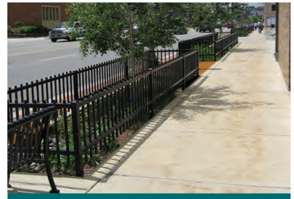
Figure 4.3.32: If grades necessitate a deep bioretention planter, then appropriate fencing should be provided around the planter as was done in this example from Lansing, MI. The Lansing design also incorporated street trees into the planters. (Source: CVC )
