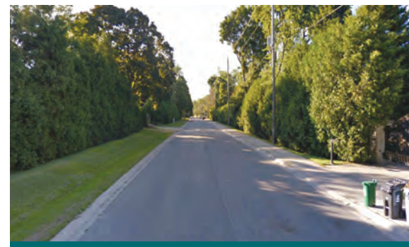
Figure 6.5.3: Low maintenance subsurface practices like perforated pipe systems or enhanced grass swales are best for areas where there is little municipal maintenance and/or high rental rates. In this picture a grass swale is used above a perforated pipe exfiltration system in Toronto, ON. (Source: CVC)
