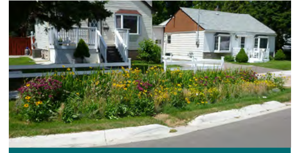
Figure 2.1.7: Boulevard bioretention units are ideally suited for road reconstruction projects upgrading residential streets with a rural cross section to an urban cross-section. This photo shows a home in the Lakeview neighbourhood in Mississauga with a planted boulevard bioretention unit. (Source: CVC)
