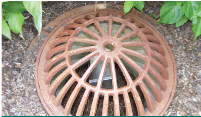
Figure 6.4.9: Properly sized grates can prevent debris from accumulating in storm sewers. Steel grates are recommended because they are more durable than plastic. (Source: Aquafor Beech)
