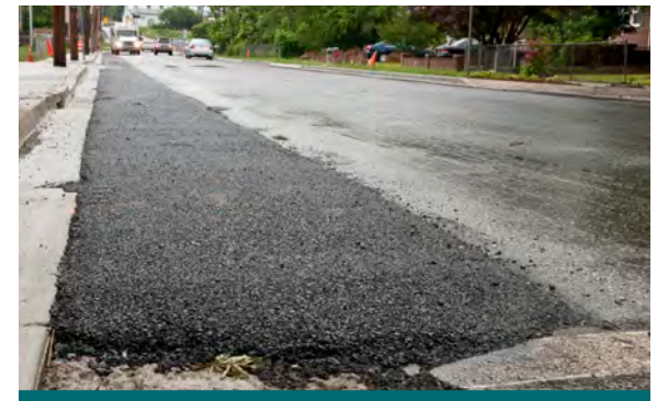
Figure 2.5.2: Porous asphalt was used to create a permeable bike lane in Edmondston, MD. As pervious asphalt can look quite similar to traditional asphalt, municipalities should track the location of permeable infrastructure to ensure that it is not re-paved in future roadwork. (Source: CVC)
