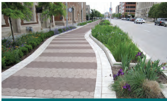
Figure 6.5.1: Bioretention planters with more elaborate landscaping may be appropriate in showcase areas where the municipality will invest in regular maintenance and beautification. The bioretention planters above are in a downtown high profile location where maintenance regularly occurs. (Source: CVC)
