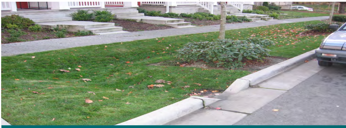
Figure 2.2.1: Enhanced grass swales have been implemented successfully throughout the United States and Canada. (Source: CVC)
