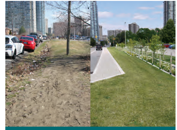
Figure 4.3.11: Before and after pictures of a residential collector, Elm Drive West in Mississauga, improved from a rural cross-section with degraded ditch to an urban cross-section with permeable paver parking laybys and sidewalk. The new design eliminated the degraded swales and improved safety for street parking. (Source: CVC)
