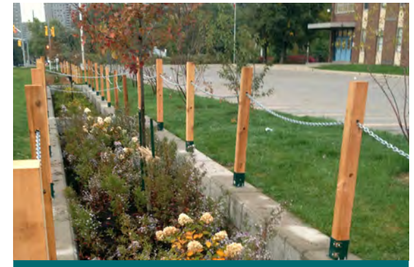
Figure 2.1.2: Bioretention planters aren't just for highly urbanized road ROWs. Planters were used to retain additional road runoff from Elm Drive in Mississauga. (Source: CVC)
