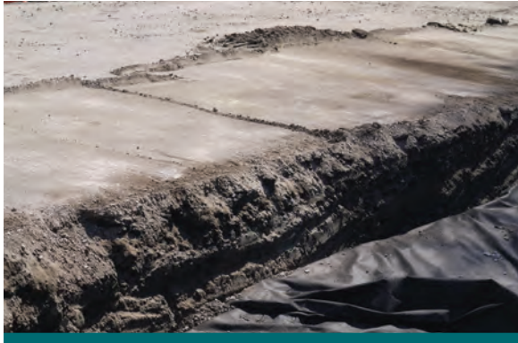
Figure 9.5.1: Sediment and dust accumulate quickly on a construction site. Daily cleanup and street sweeping were worked into the schedule at the Lakeview Project. (Source: Aquafor Beech)
