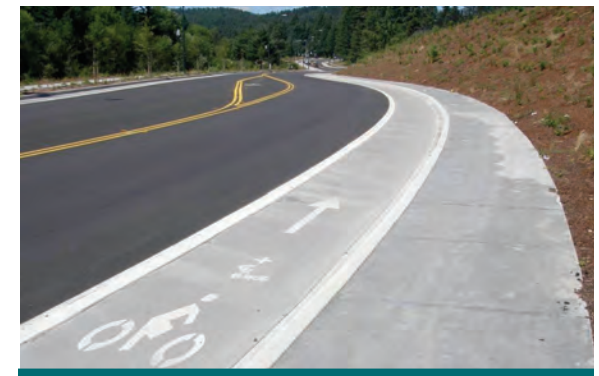
Figure 4.3.12: Pervious concrete bike lane and sidewalk in, City of Olympia, WA. (Source: City of Olympia)
