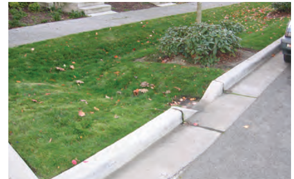
Figure 6.4.7: Consider existing trees, parking spaces and other ROW features when selecting inlet type and location. (Source: CVC)
