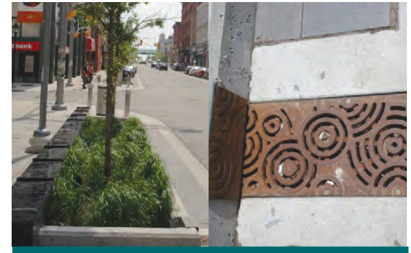
Figure 4.3.31: City of Kitchener incorporated bioretention planters into their main commercial street, King St. The design incorporates seating and trench drains with decorative grating to take runoff from the street. (Source: CVC)
