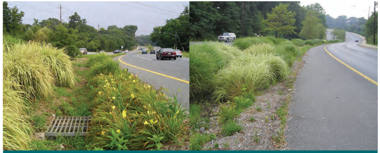
Figure 4.3.28: Bioswale incorporated into the median of an Arterial Road in Adelphi, MD. The plantings were kept to two or three attractive yet low maintenance plant species. (Source: Low Impact Development Center)
