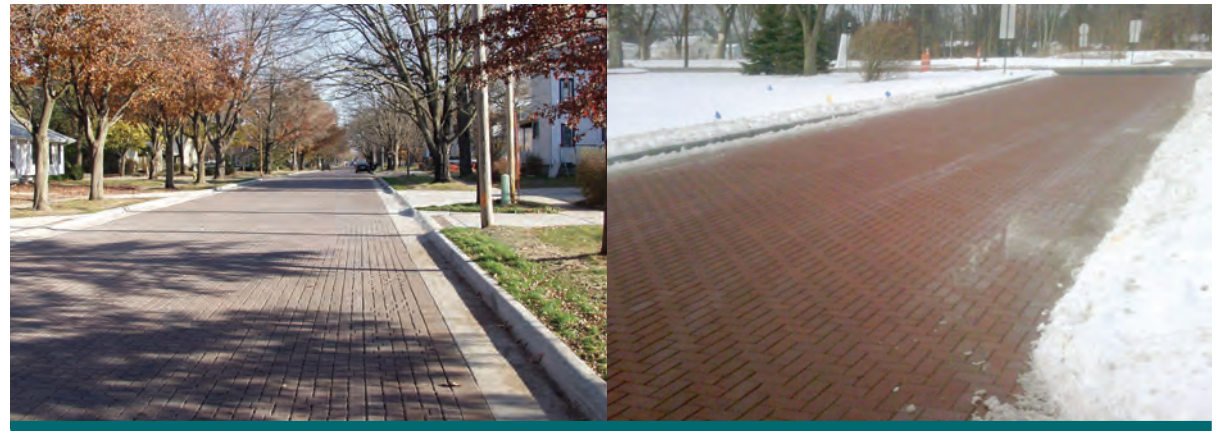
Figure 4.3.7: Permeable pavers used from curb to curb in Charles City, IA (left) and New Albany, OH (right). There are many examples of permeable pavement for the full road within cold climate regions of the US. Snow can be ploughed from permeable pavement as with any other pavement. After ploughing remaining snow can melt immediately into the permeable surface thereby reducing the use of deicers. (Source: ICPI)
