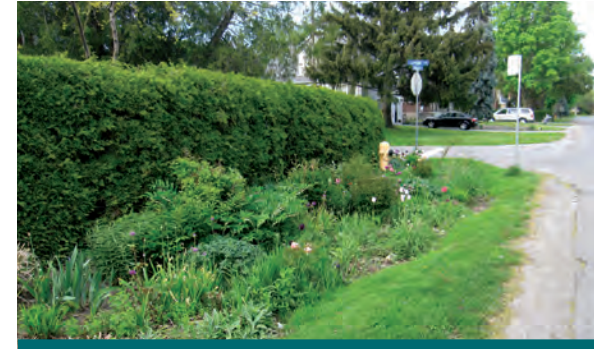
Figure 4.3.4: While many homeowners of this Toronto neighborhood have kept their enhanced swales as grass, a few have turned their swales into gardens that increase stormwater treatment and infiltration. Note that only low growing vegetation was used to avoid encroach on street corner sight lines. (Source: CVC)
