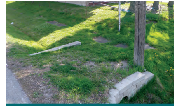
Figure 4.2.2: Unmaintained property access points that cross the conveyance path of the ROW may not be identifiable on background materials. (Source: Aquafor Beech)
