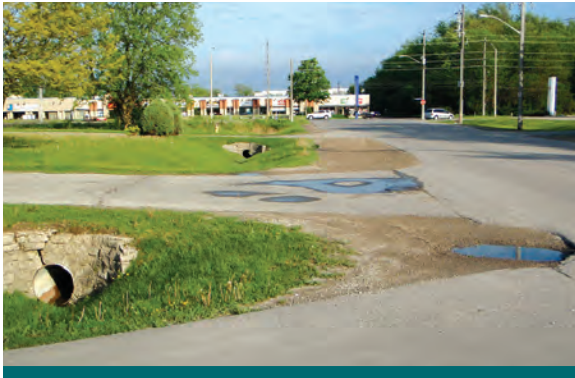
Figure 4.3.14: Local industrial road. (Source: Aquafor Beech)
