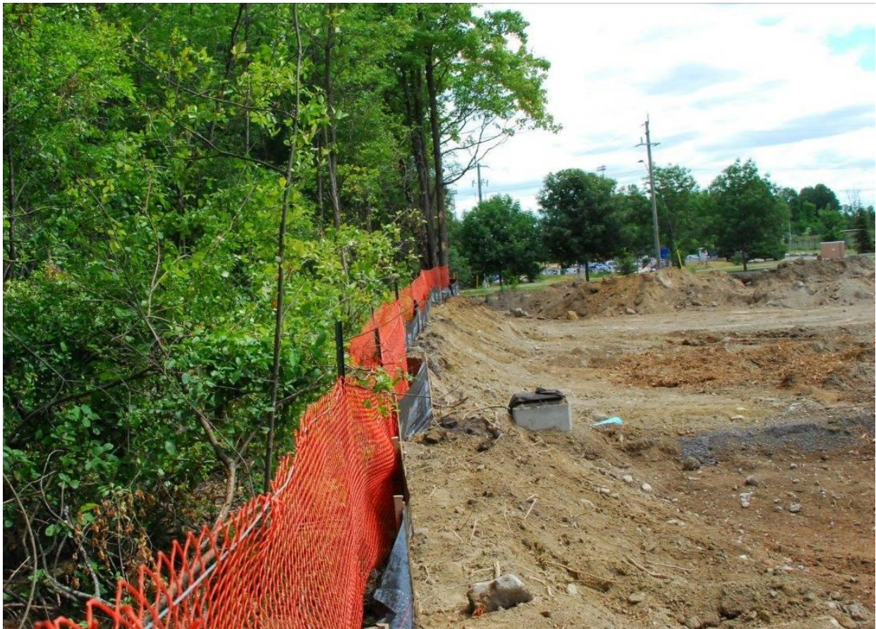
5: Properly installed and maintained fencing protects a natural area from adjacent site alteration work.
