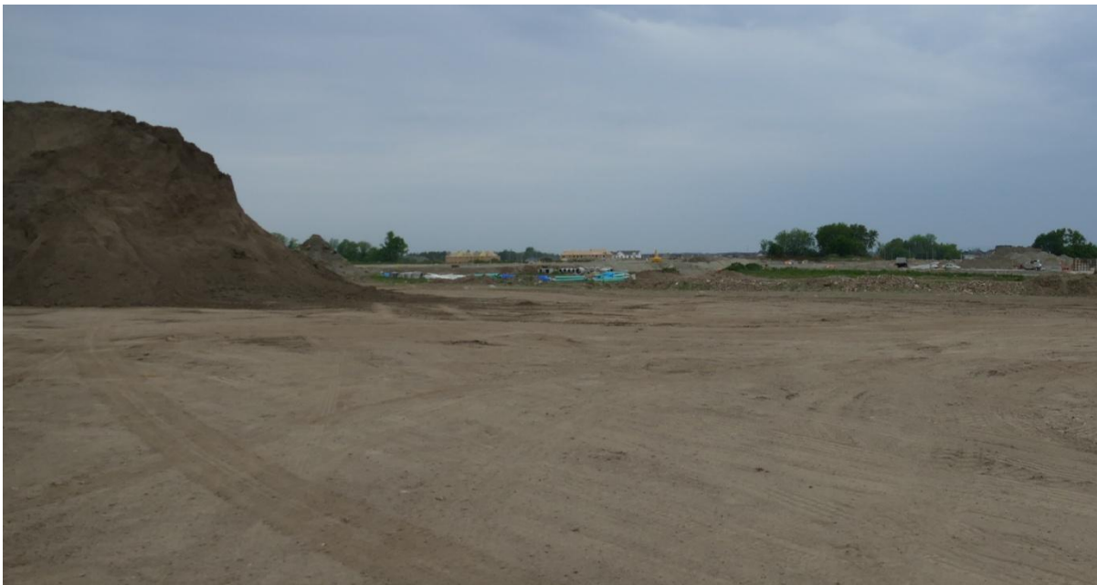
3: Site preparation in advance of development, showing stockpiled topsoil and exposed subsoil.
